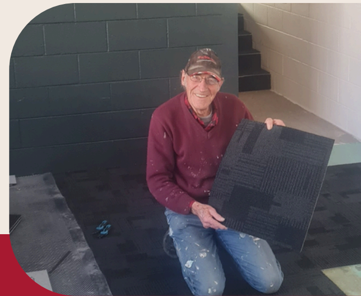
Devonport Chaplaincy Office Project, TAS
